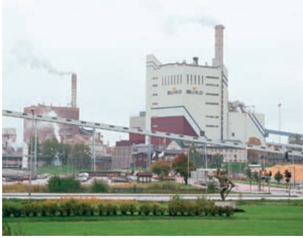
Figure 4: CHP in pulp and paper application using VST-SE steam conditioning valve
