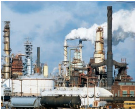
Figure 6: VST-SE for more reliable and efficient operation at petrochemical facilities.
